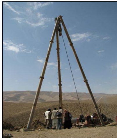
Sinking a 100 metre deep well in a dry and parched land.
