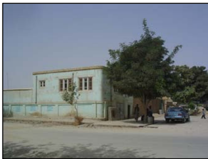
Outside New Office in Dawlatabad
