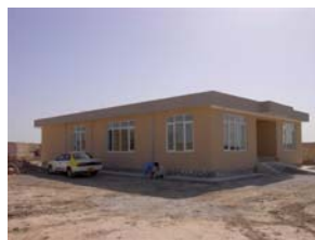
The Completed Clinic
